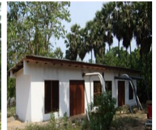
Reconstruction of Visvamadu lift irrigation scheme in Mullaitivu District
