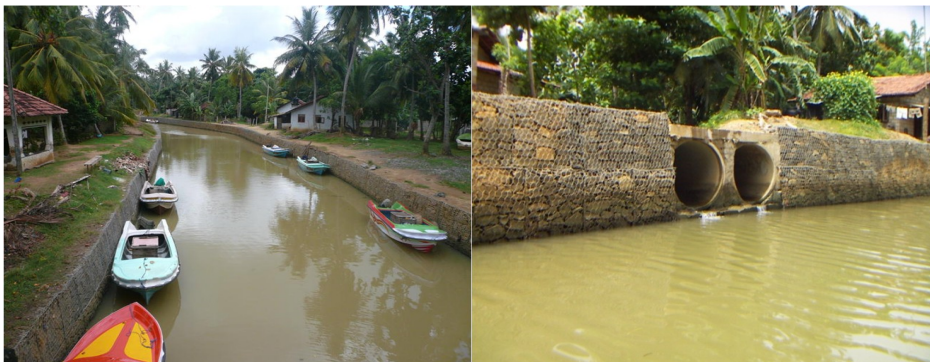
Rehabilitation of Hamilton Canal
