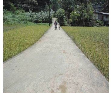
Construction of "Kanuwatta" agrarian road at Wiguhumpola -
