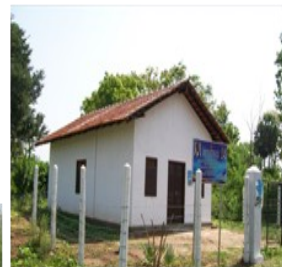
Reconstruction of Common Hall at Paddikudiiruppu in Vavuniya District
