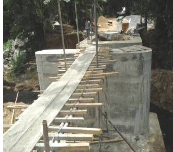
Construction of Weewala bridge at Narangaspitiya ( 2nd stage)
