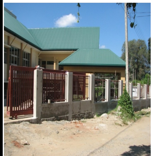
Newly constructed Hotel School Building Kandy
