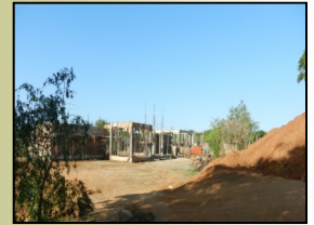
Construction of main entrance complex at Dry zone Botanic Gardens, Hambantota
