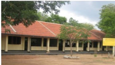
Reconstruction of School building at Kilinochchi Hindu Primary Vidyalaya
